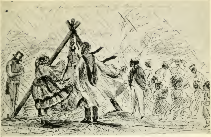
LAYING THE FOUNDATION STONE OF BIMLIPATAM CHURCH BY THE REV. J. GRIFFITHS.
