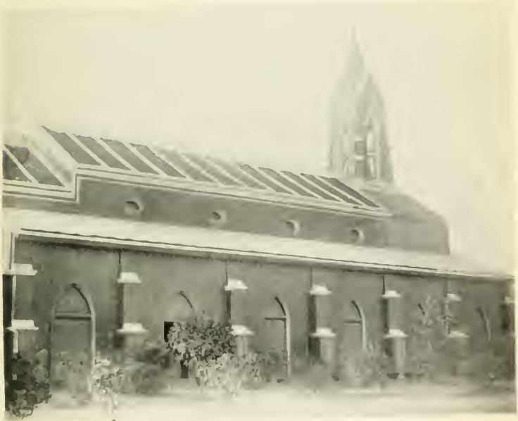
ST. PETER'S CHURCH, BIMLIPATAM.
