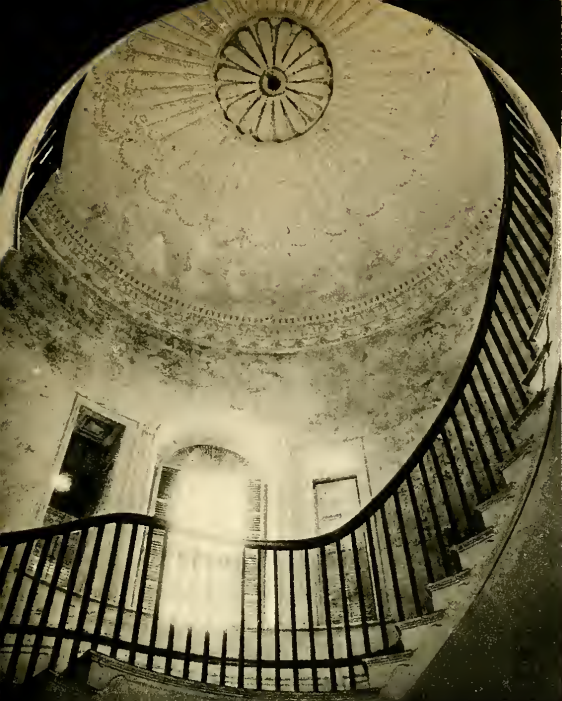
STAIRWAY JOSEPH MANIGault HOUSE (1790-97) CHARLESTON Designed by Gabriel Manigault
