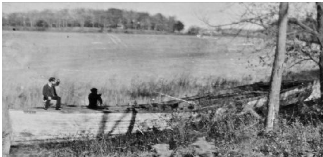
The barge Mermaid , formerly the Governor Ramsey , was left to rot on the north shore of Shady Isle on Upper Lake Minnetonka. MHM hopes she was towed into the lake and sunk (Reserve Album 111 #41, Minnesota Historical Society).
